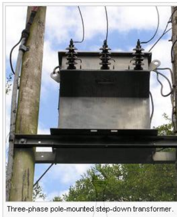
Three-phase pole-mounted step-down transformer.
