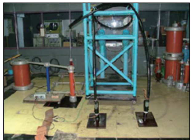
Figure 10: Show the circle of line connection which is using gas SF 6 to be insulation testing for finding the partial discharge value in the high voltage cable in the side of 24 kV
