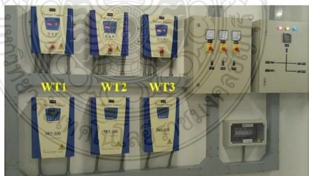
**Figure 3.7** Grid-Connected Inverters of THUNYA-5-kW HAWTs in Electrical Control Room of DETC
