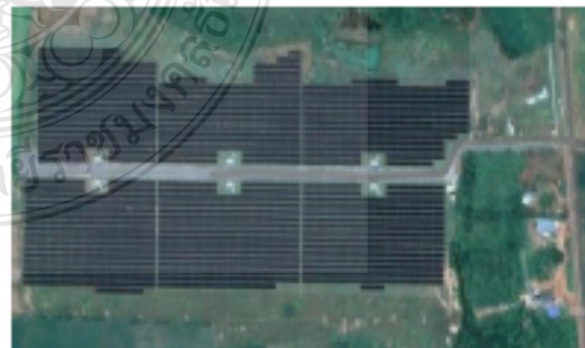
Fig. 1. PV power plant [17]
