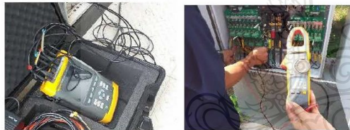
(a) Power meter (b) Clamp meter
