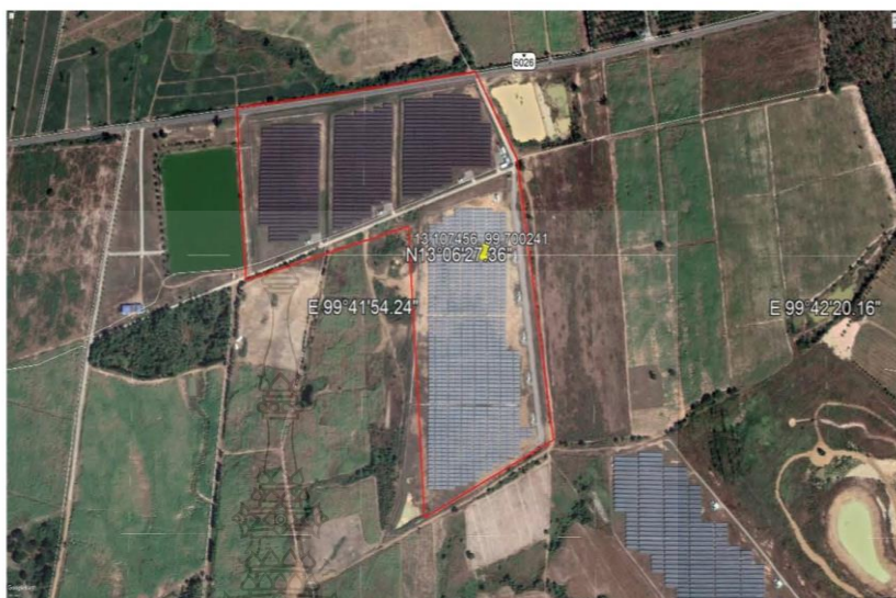
Figure 3. Location of the implementation of the PV power plant [22].
