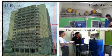
Fig. 11, building 13 Floors Control room of EERU and energy recorder are installed
