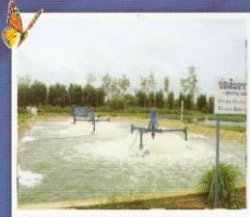
Design, construction, installation and commissioning wastewater treatment plant, capacity 1,200 cu.m./day
